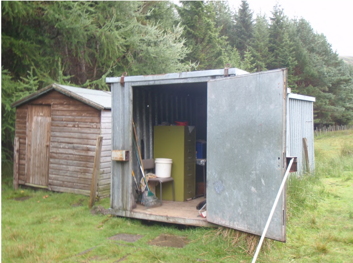
Figure 3. – Existing cabin and storage shed
